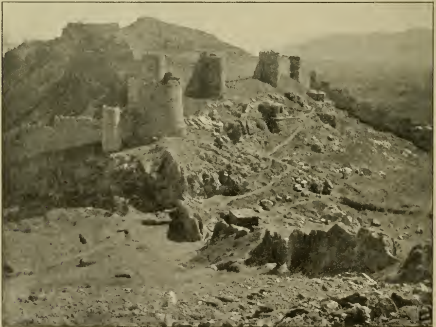
FIG. 240. Outer wall of Kabul, capital of Afghanistan.
